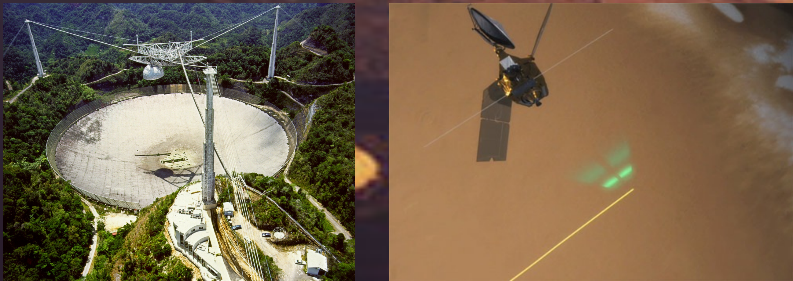
Arecibo Observatory provides S-band (12.6 cm) radar observations of Mars SHARAD, the Shallow Radar on Mars Reconnaissance Orbiter, emits a 25–15 MHz signal.
